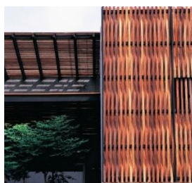
Figure 3. Applying regional resources to finish the roof and elevations
