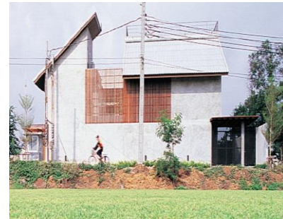
Figure 4. 45° to 55° high roof angle for rain drainage
