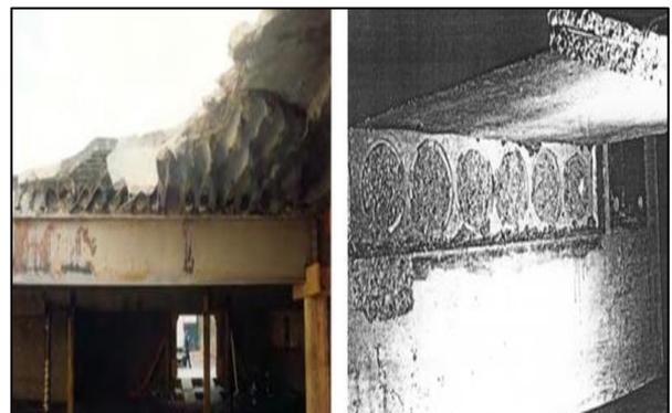
**Figure 1.** Failure of Hollow-Core in the 1994 Northridge earthquake [8]
