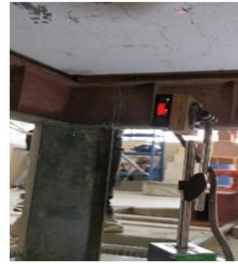
Figure 8. Deflection gage sensor
