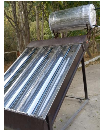
Figure 1. Real case of compound parabolic collector (CPC) which is modeled in the simulations
