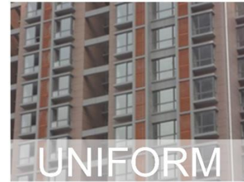
Figure 7. Uniform outdoor AC unit arrangement
