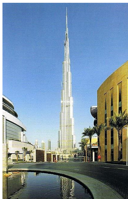
Figure 2. Khalifa Tower in Dubai
