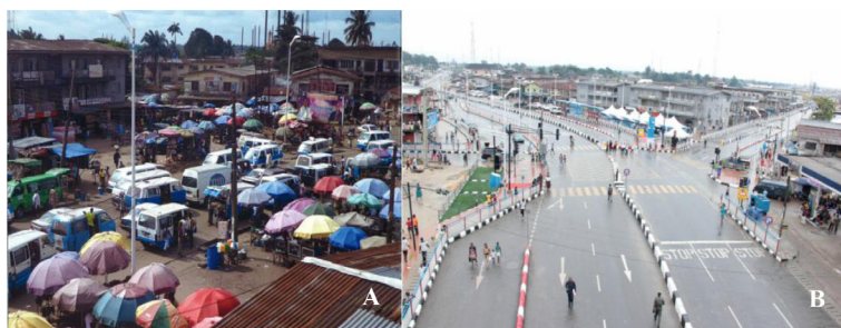
Figure 1: Drone view of Enerhen road junction network. A – Failed network, B – Newly constructed network.
