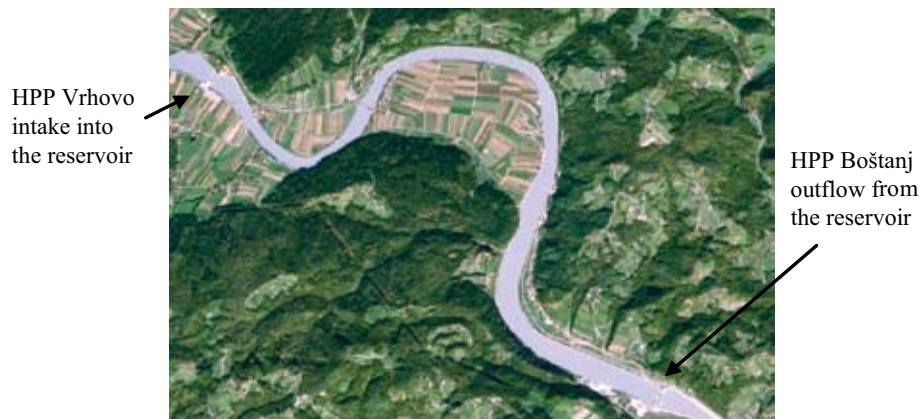
Figure 1: Water-storage reservoir of the HPP Boštanj on the Sava River.
