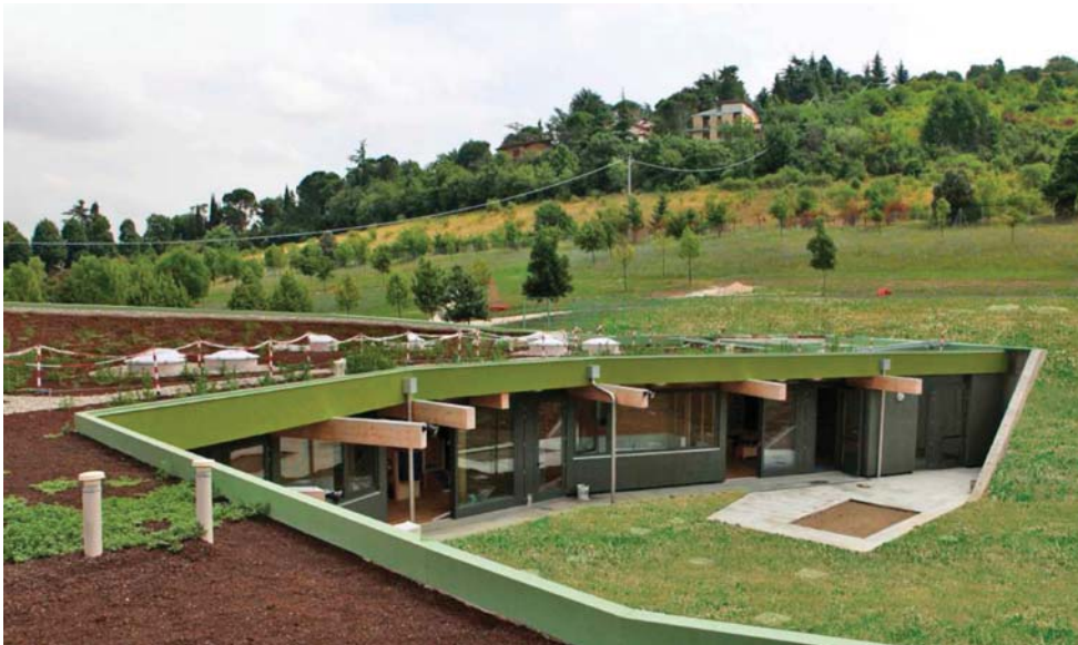
Figure 6: A green roof can contribute toward the increase of thermal inertia. A green roof is an element of integration with the environment and of microclimatic control. It has a thermal transmittance U = 0.20 \text{ W/m}^2\text{K} and a phase displacement of 10 hours. Day nursery, Gainaido in Bologna (HGT = 2259), 2009 Tasca Studio.
