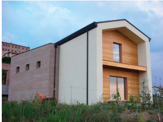
Figure 9: Montiano (FC), Italy, HGT = 2356. Passive residential building. The regular and compact shape helps the energy control; the orientation and limited size of clear surfaces limit summer overheating.
