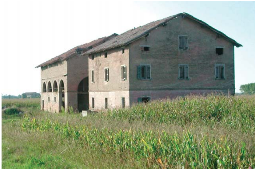
Figure 3: A traditional rural building in Italy, Emilia Romagna, HGT = 2560, the monthly average outside temperature during the winter heating period is of 5.96°C, characterized by massive materials and protection elements from solar radiation. The compact volume provides a favorable ratio S/V = 0.6 (ratio between dispersant surfaces and heated volume).
