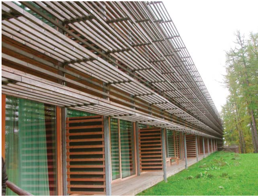
Figure 8: Shaded surface in a bioclimatic hotel. Class A Klimahouse [19]. Vigilius Mountain Hotel, Lana – Bolzano (HGT = 2791; monthly average outside temperature during the winter heating period 4.73°C), Italy, arch. Matteo Thun.
