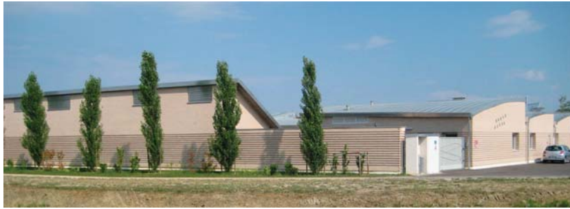
Figure 2: 'Lama Sud' school – Ravenna, Italy. Its massive envelope assures high performances also in warm climate context. HGT = 2,227 and the monthly average outside temperature during the winter heating period of 6.62°C, a climate characterized by cold winters and hot summers.
