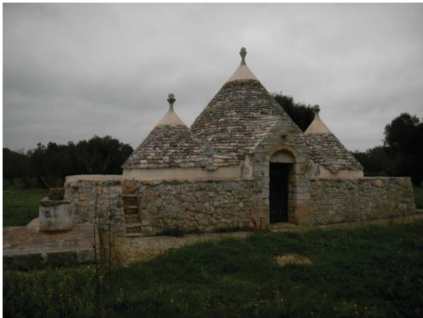
Figure 1: The massive envelope assures high performances in terms of thermal inertia in a warm climate context. 'Trullo', a traditional construction in Southern Italy, Puglia (HGT = 1100; monthly average outside temperature during the winter heating period of 10.7°C).
