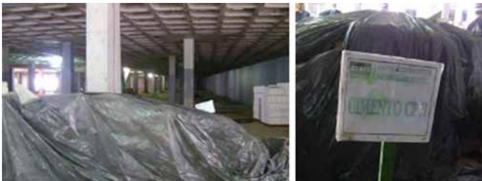
Figure 13: Storage of protected cement bags.
