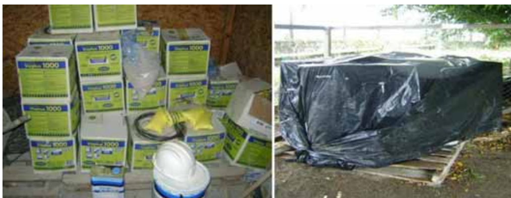
Figura 14 – Storage of waterproofing materials.
