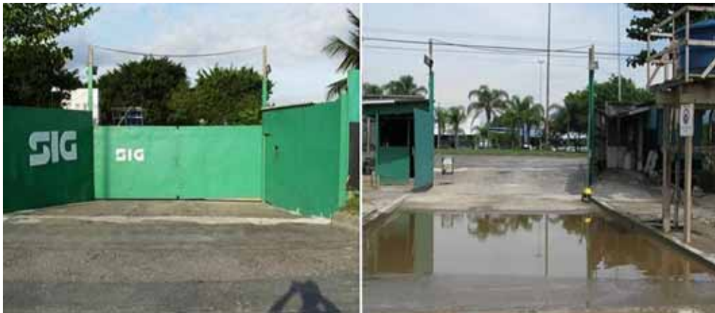
Figure 4: Site entrance and wheel wash.
