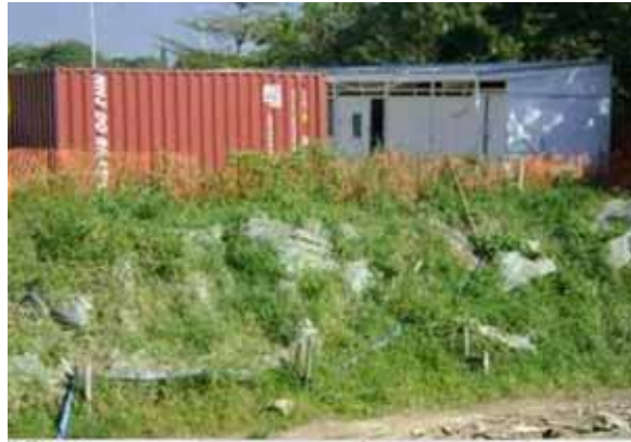
Figure 2: Embankments protected by vegetation.
