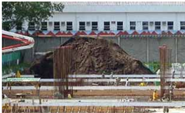
Figure 12: Excavated material that was reused for landfill.
