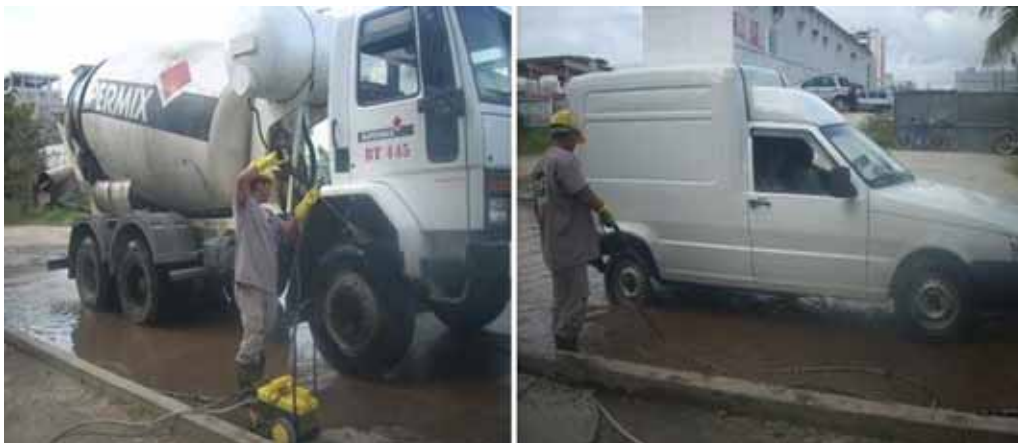
Figure 5: Auxiliary water pump.
