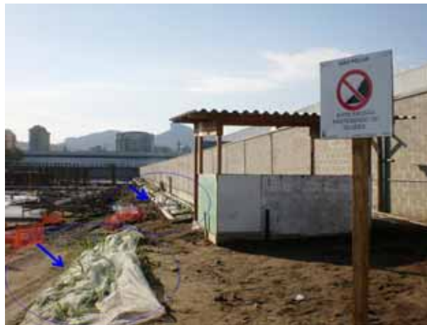
Figure 1: Embankments protected to avoid erosion.
