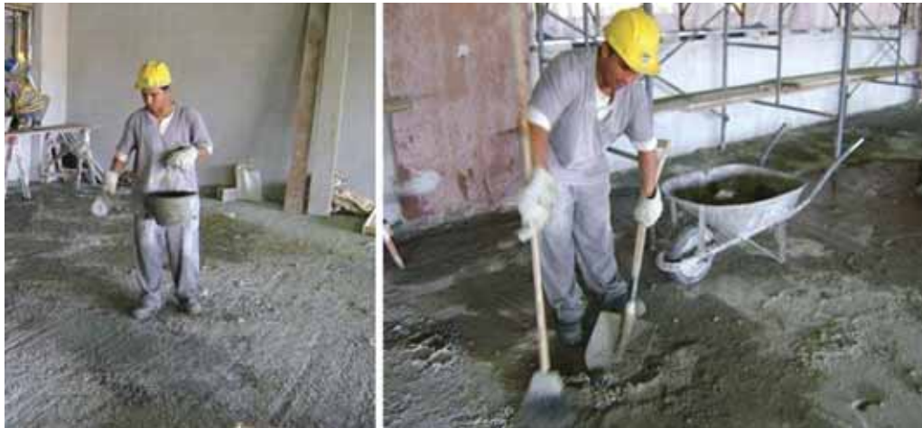
Figure 3: Sedimentation control by soaking and sweeping of the construction site.
