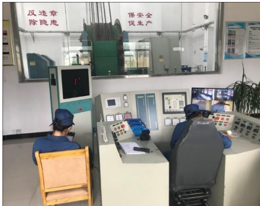
Figure 1. The console of the hoist room
