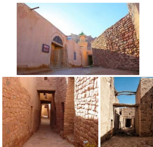
Figure 5. Architectural features of Al-Ula old-town [3]
