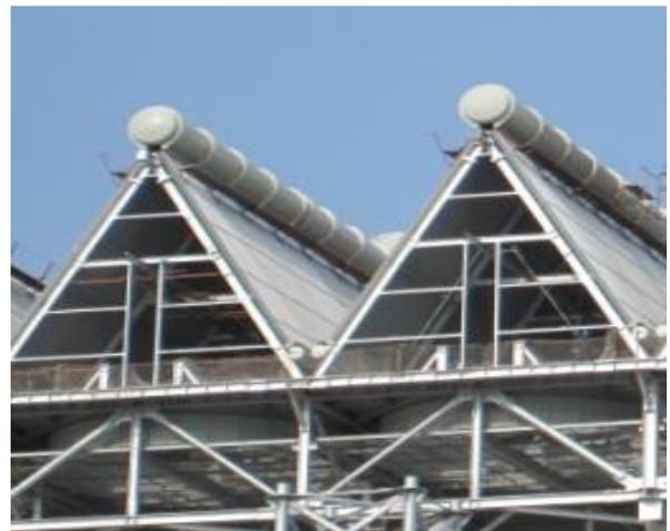
**Figure 1.** Schematic representation of an A-frame condenser cell
