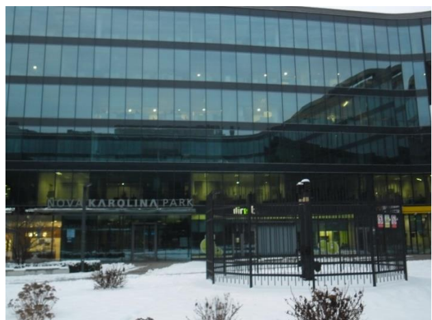
Figure 7. Protection of Nova Karolina Park at Ostrava by means of gas drainage borehole
