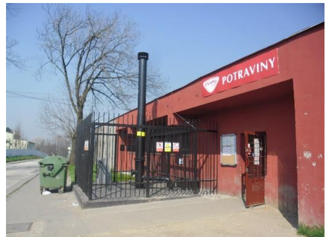
Figure 4. Building of shopping centre protected by means of gas drainage borehole Na Liščině street, Ostrava- Hrušov
