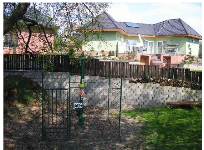
Figure 5. Protection of a family houses at Ostrava -Muglinov in the area of decommissioned prospect
