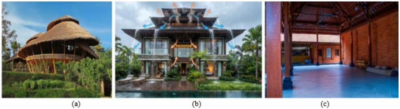
Figure 2. Balinese vernacular passive-design elements documented in the study context: (a) open pavilion with opposing openings supporting cross-ventilation; (b) elevated roof volume with high-level ventilation; (c) locally sourced envelope materials and shaded transitional space Source: Hotel official documentation, 2026.
