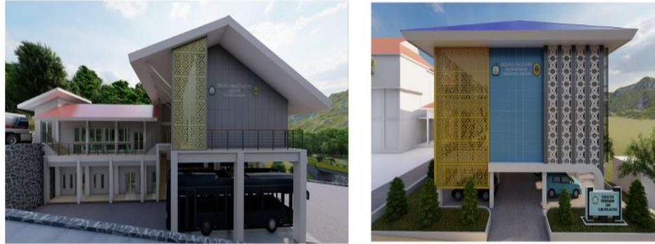
Figure 11. New campus buildings under construction, adopting the nutmeg-clove sunscreen language
