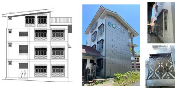
Figure 7. Type B laboratory sunscreen technical drawing showing density variation, internal zoning response, and Aluminium Composite Panel (ACP) module assembly
