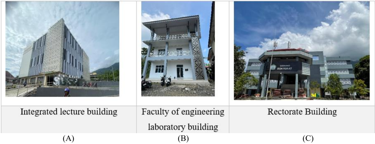
Figure 3. Typologies of nutmeg-clove-inspired Aluminium Composite Panel (ACP) sunscreen systems at Khairun University: (A) Type A academic, (B) Type B laboratory, and (C) Type C administrative buildings
