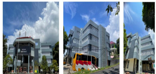
Figure 8. Type C administrative sunscreen: Nutmeg-clove motif with lower porosity and stronger institutional facade order in the Rectorate Building
