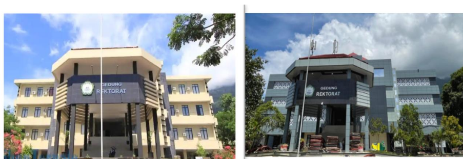
Figure 10. Rectorate Building before and after the installation of the Type C nutmeg-clove-inspired Aluminium Composite Panel (ACP) sunscreen system
