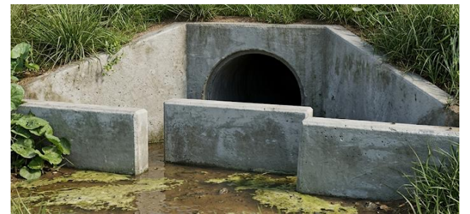
Figure 6. Photograph of a baffle-wall energy dissipator illustrating the internal energy dissipation
