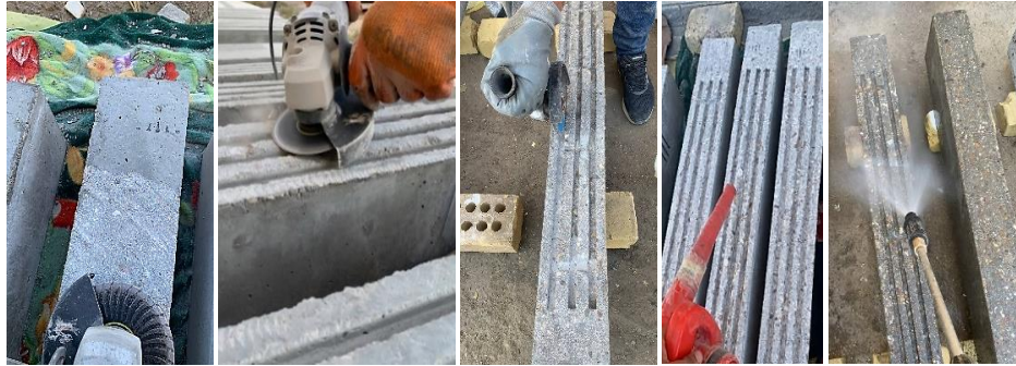
Figure 5. Preparation, roughing, cleaning, and washing process
