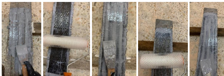
Figure 7. Externally bonded reinforcement on groove (EBROG) strengthening process
