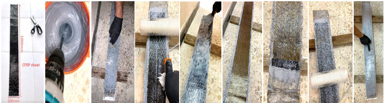
Figure 6. Externally bonded reinforcement (EBR) strengthening process
