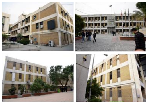
Figure 8. Real pictures of the building
