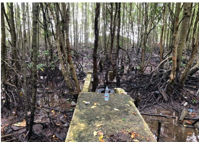
Figure 2. Disconnected access infrastructure at the Dumai city mangrove tourism
