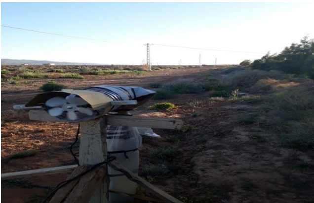
Figure 1. Earth to air heat exchanger inlet and outlet
