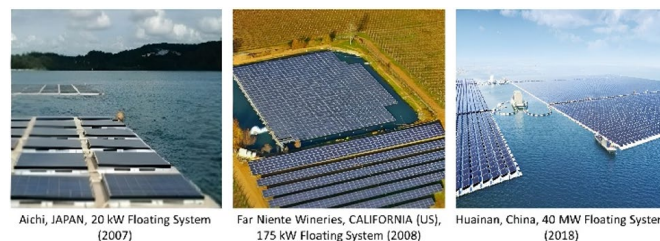
Figure 2. The first FPVS (Aichi, Japan), the first commercial FPVS (California, USA), and the world's largest FPVS (Huainan, China)
