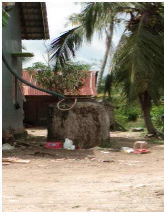
(a) The storage tanks used by the first generation were made of cement
