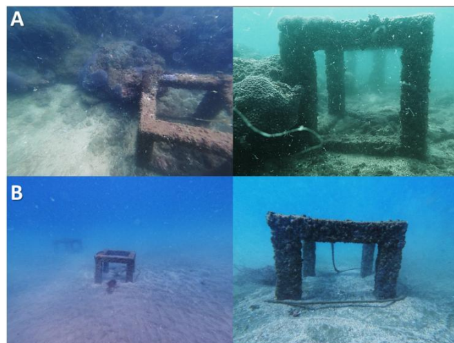
Figure 4. Documentation of artificial reef placements at Damas Beach showing two contrasting conditions — (A) Artificial reef structures placed too close to natural coral reefs, potentially causing ecological interference; (B) Artificial reef structures placed in barren sandy areas far from existing coral reefs, reducing their effectiveness as alternative habitats and buried in sediment
