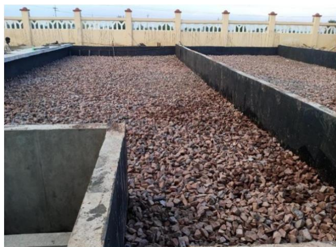
Figure 6. Preparation of bed materials in CW
