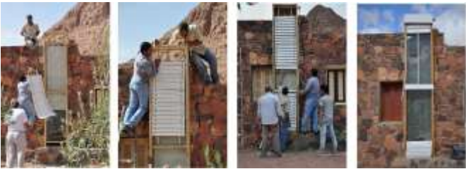
Figure 9. Installing the TW components and securing the operational mechanism [69]
