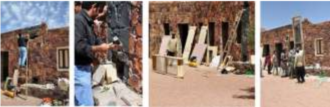
Figure 8. The entire TW installation procedure, from cutting the vents to installing the wall's components [69]
