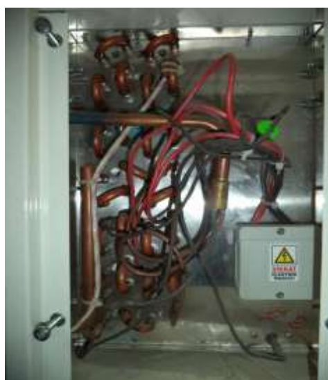
Figure 12. Pipes connections of evaporator
