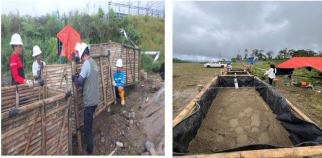
Figure 4. Wetland installation settings and materials filling
