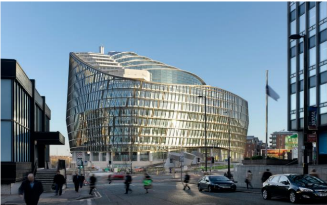
Figure 2. One Angel Square Note: The double skin can be seen on the façade, thus generating adiabatic cooling, which is based on evaporating the water that resides in the air by Hopkinson et al. [48].
