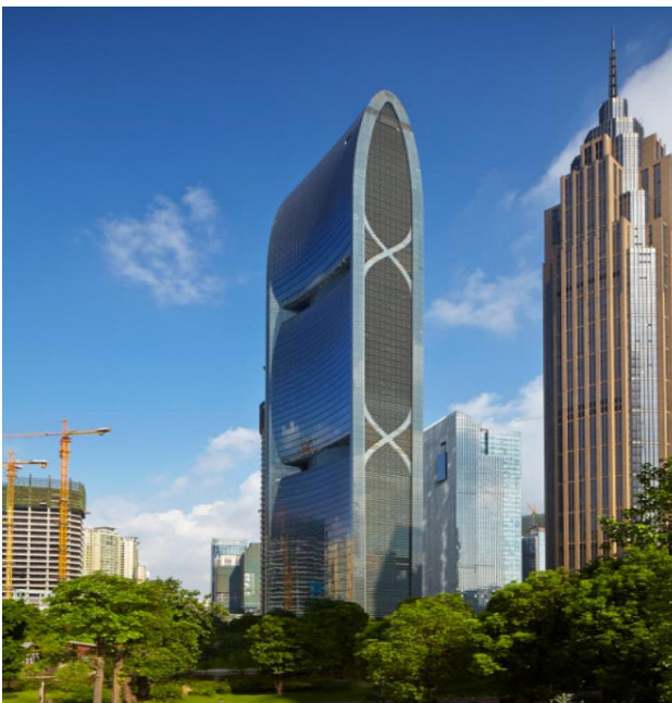
Figure 3. Tower Pearl River Note: A double-skin curtain wall can be seen on the facade, with a modern structuring system by Zhang [49].
