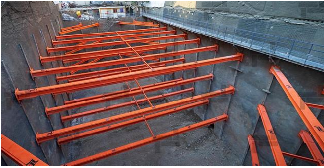
Figure 1. Stabilization of pit walls using strut method in Sepidar project [3]
