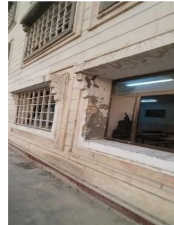
Figure 6. Condition of the paint finishing materials (WPai+GT1) on the window frames of the façade of Asma Bent Abi Bakr School
