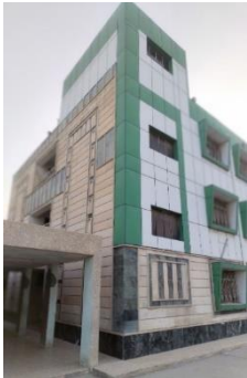
Figure 14. Condition of the finishing materials (marble, stone, and aluminum panels) on the exterior facade of Al-Shaheed Qahtan Ali Al-Lami School
