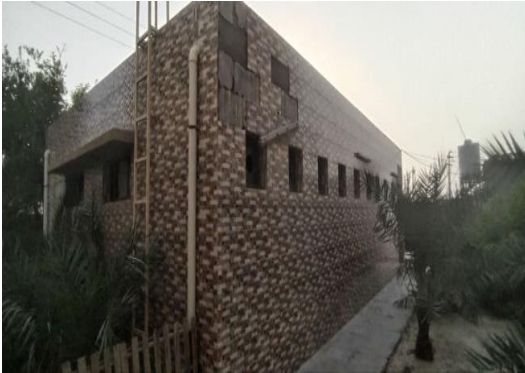
Figure 15. Condition of the ceramic finishing materials on the exterior of the restrooms at Al-Shaheed Qahtan Ali Al-Lami School
