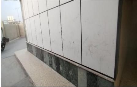
Figure 16. Condition of the ceramic finishing materials on the exterior of the restrooms at Al-Shaheed Qahtan Ali Al-Lami School
