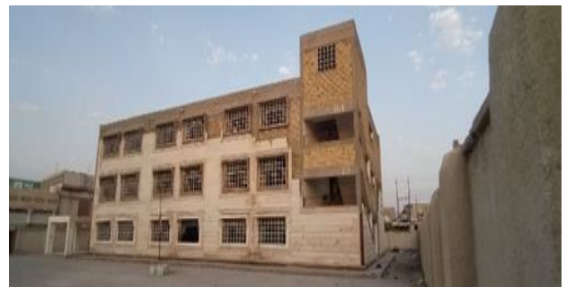
Figure 5. Condition of the natural stone finishing materials (ST1) in the façade of Asma Bent Abi Bakr School
