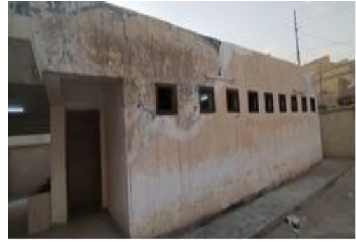
Figure 9. Condition of the paint finishing materials (WPai+GT1) on the sanitary façade of Asma Bent Abi Bakr School
