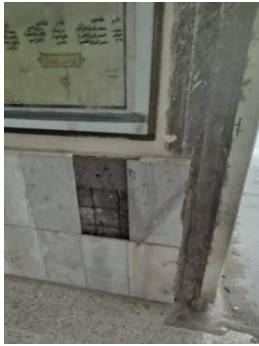
Figure 8. Condition of the finishing materials on the façade of Asma Bent Abi Bakr School, specifically the white marble (MAT3)
