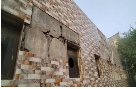
Figure 16. Condition of the ceramic finishing materials on the exterior of the restrooms at Al-Shaheed Qahtan Ali Al-Lami School
