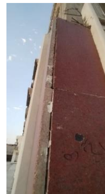
Figure 7. Condition of the red granite finishing materials on the façade of Asma Bent Abi Bakr School (GRT3)
