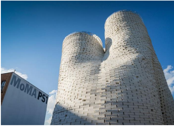
Figure 2. Tower of "grown" bio-bricks by The Living opens at MoMA PS1 Source: Frearson [19]
