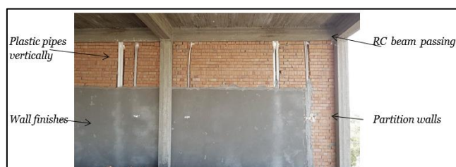
Figure 5. Vertical services pipes hidden through wall finishes (Commercial building/Babil-Iraq)
