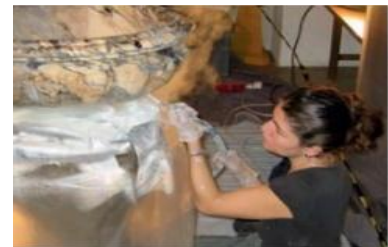
Figure 4. A portable steam cleaner used to clean decorative marble pieces [29]
