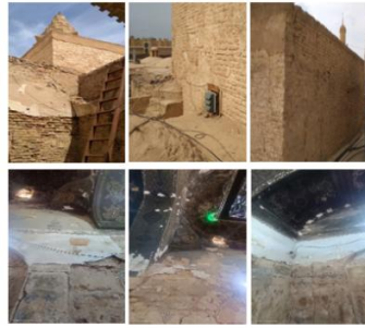
Figure 7. Natural and unnatural deterioration factors (neglect, humidity, and the effect of candles)
