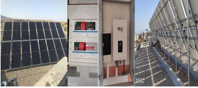
Figure 2. Components and configuration of the solar panel system
