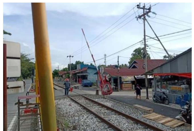
Figure 1. Illegal crossing without guard post
