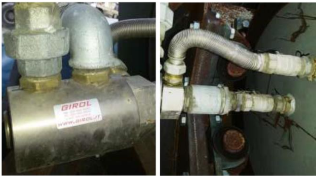
Figure 10. Rotary coupling for the distribution circuit of the fluid in the shaft
