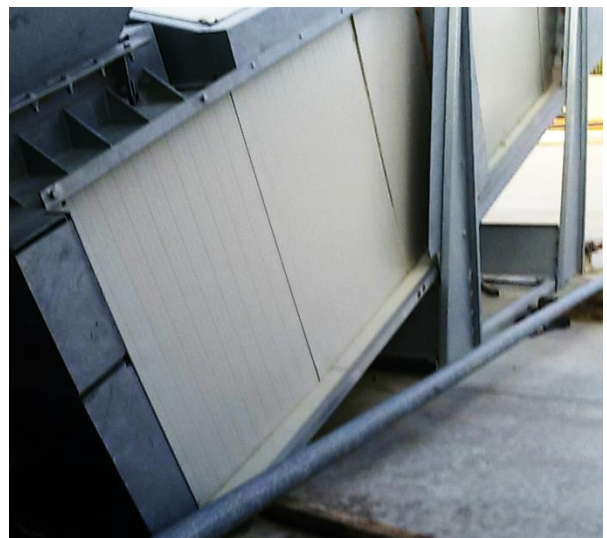
Figure 13. Cover insulating sandwich panels for the outer tub to the auger
