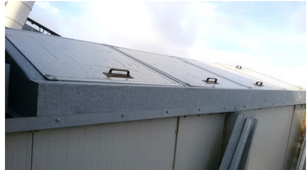
Figure 12. Cover insulating sandwich panels on the sloped roof
