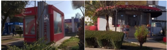
Figure 16. Elements of the kiosk group
