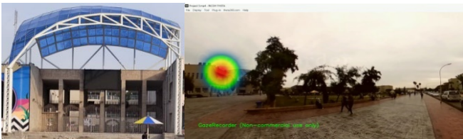
Figure 15. Student center dome
