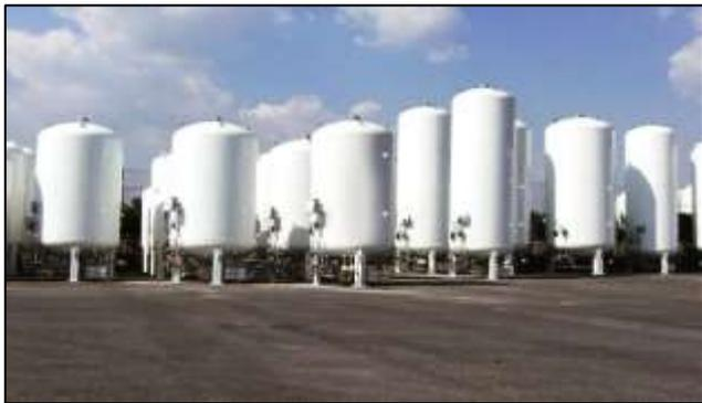
**Figure 1.** CO<sub>2</sub> storage tank with steel walls
