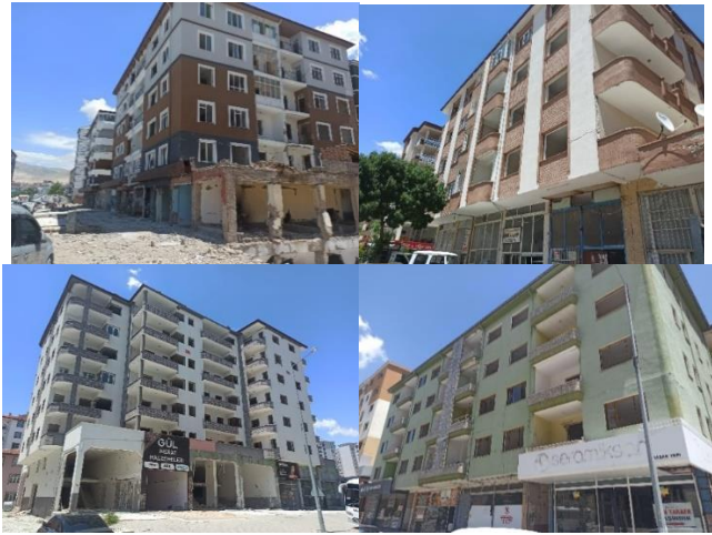
Figure 5. Examples of severely damaged and evacuated buildings in Sahinali Neighborhood (Original)
