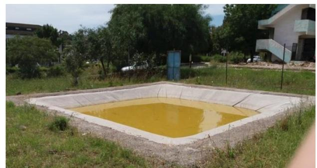
Figure 2. Real solar pond constructed at Annaba University ( $7\text{ m} \times 7\text{ m} \times 2\text{ m}$ )
