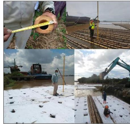
**Figure 4.** The bamboo was used as a mat and pile for preloading the base structure before monitoring the works
