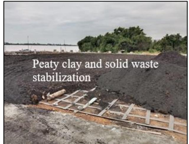
**Figure 13.** Stabilization of the peaty clay using solid waste from the biomass power plant at the final stage of preloading
