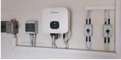
**Figure 3.** Rooftop PV power plant inverter installation
