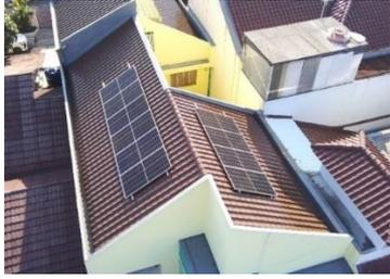
**Figure 2.** Installed rooftop PV power plant system
