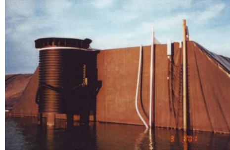
**Figure 17.** Poles on which RTD sensors and sampling tube were attached
