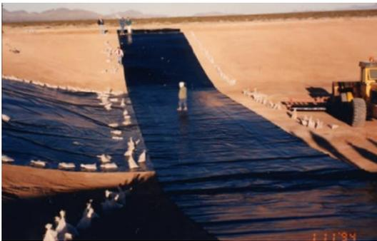
**Figure 7.** Flexible polypropylene geomembrane liner installation
