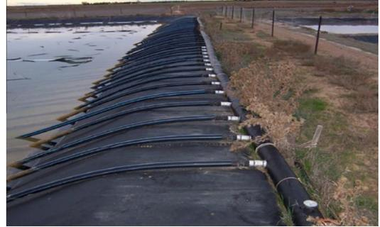
**Figure 14.** Heat extraction tubes connected to polyethylene manifold pipes
