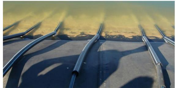
**Figure 15.** Heat extraction tubes insulated and inserted in larger plastic tubes
