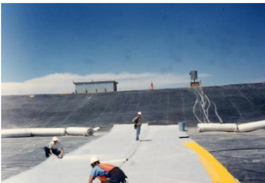
**Figure 8.** Geotextile installation
