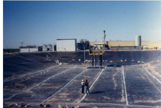
**Figure 9.** Liner system installed
