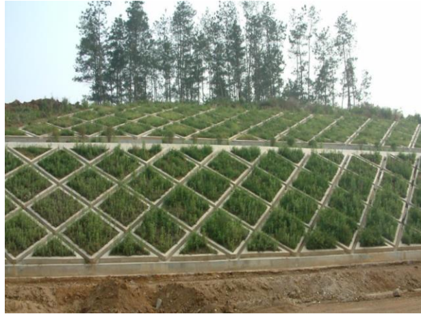
Fig.2.Effect drawing of frame beam slope protection
