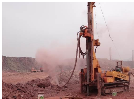
Figure 10. Reverse circulation drilling effect on site
