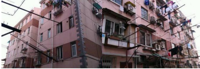
(a) North facade (b) South facade
