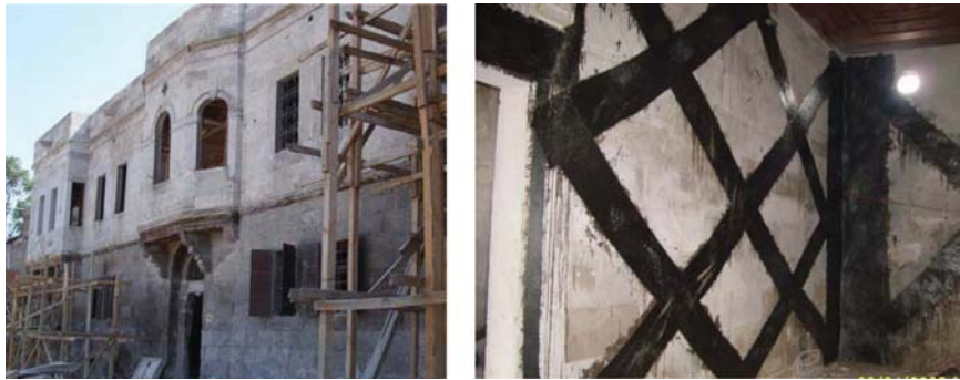
Figure 11: Front wall external view and CFRP application on the inner face.
